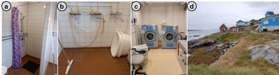
Figure 18. Service house in Itilleq. Greywater from (a) showers, (b) washing and (c) laundry facilities is (d) discharged to the sea through a pipe, September 2024.
