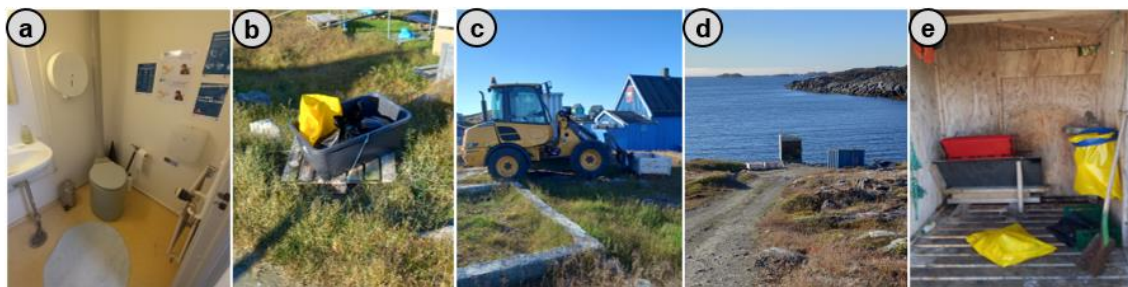
Figure 15. Sanitation in Itilleq: (a) dry toilet in the service house, (b) bags stored outside the household, (c) tractor with a shovel to pick up the bags, (d) latrine disposal site with a sea view, and (e) latrine disposal ramp, September 2024.
