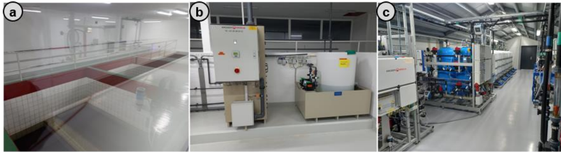
Figure 10. (a) Sand filters and (b) NaOCl dosing station at the Sisimiut WTP, August 2024. (c) View to the inside on the Itilleq WTP, September 2024.
