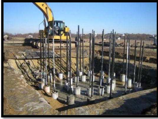
Figure 148 - Piles driven into mountain (Earth Systems)
