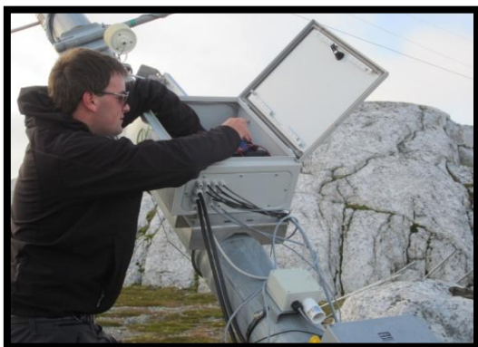
Figure 188 - Electrical installations on 1601 mast
