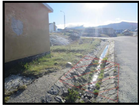
Figure 118 - Water trench behind warehouse
