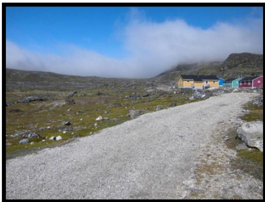
Figure 128 - Critical turn requires leaving the gravel road
