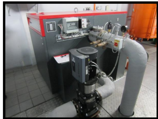
Figure 157 - Electric boiler
