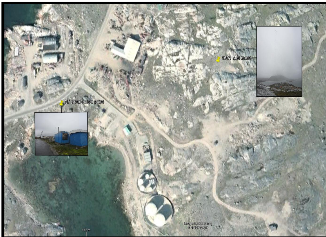
Figure 90 - Connection point and met mast site (Google Earth)
