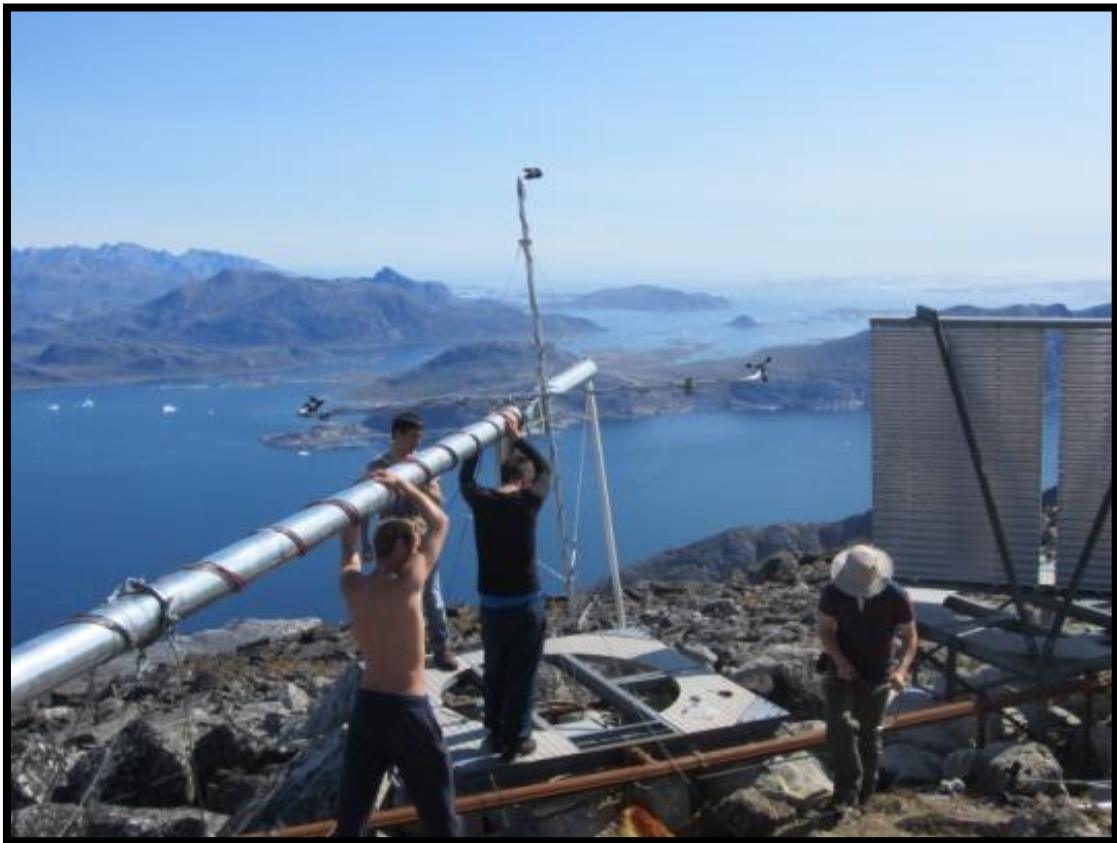
Figure 190 - Balancing the met mast at TREF
