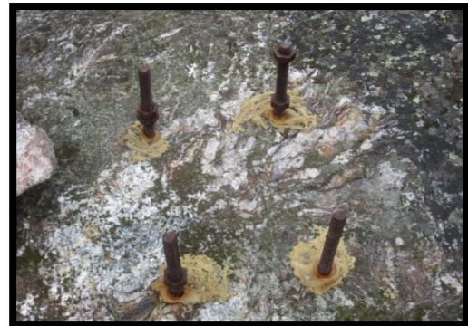
Figure 64 - Foundation of the 04283 Nanortalik Weather Station
