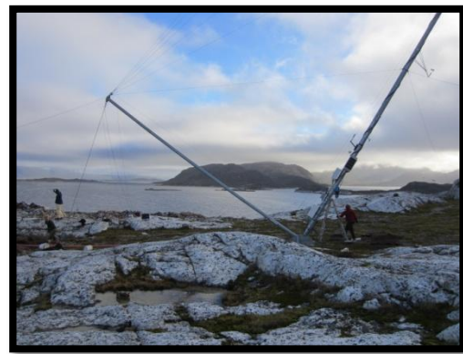
Figure 189 - Erecting the met mast
