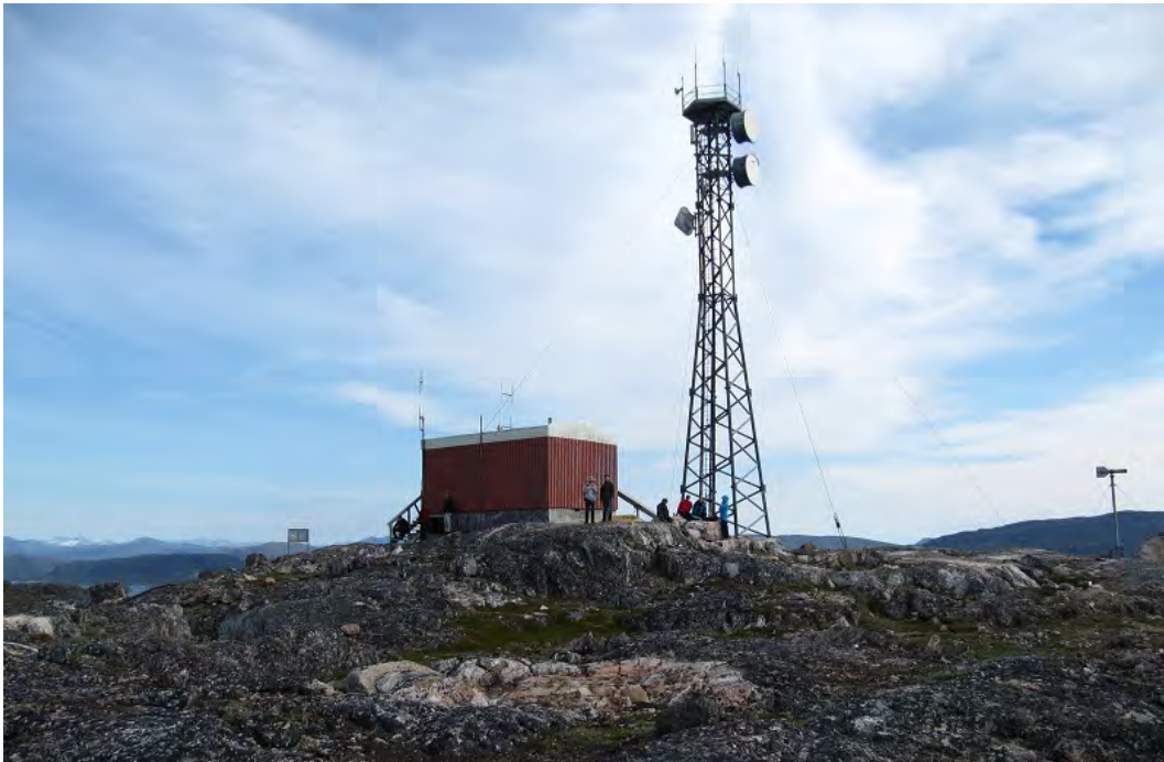
Figure 11: Telecommunication tower close to the north wind farm site.
