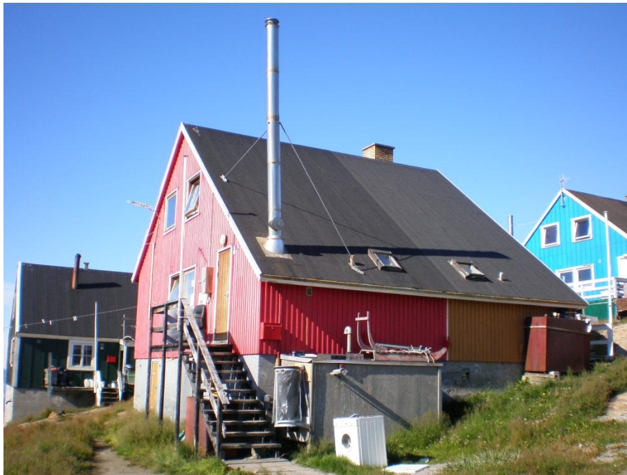
FIGURE 8: A TYPICAL DESIGN FOR A FAMILIAL GREENLANDIC HOUSE, EQUIPPED WITH AN INDIVIDUAL OIL BOILER.
