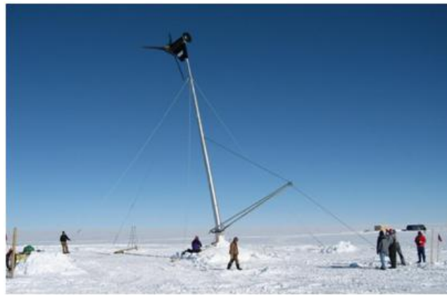
Figure 15: Putting up the Proven Wind Turbine at the Summit Station, Greenland.
