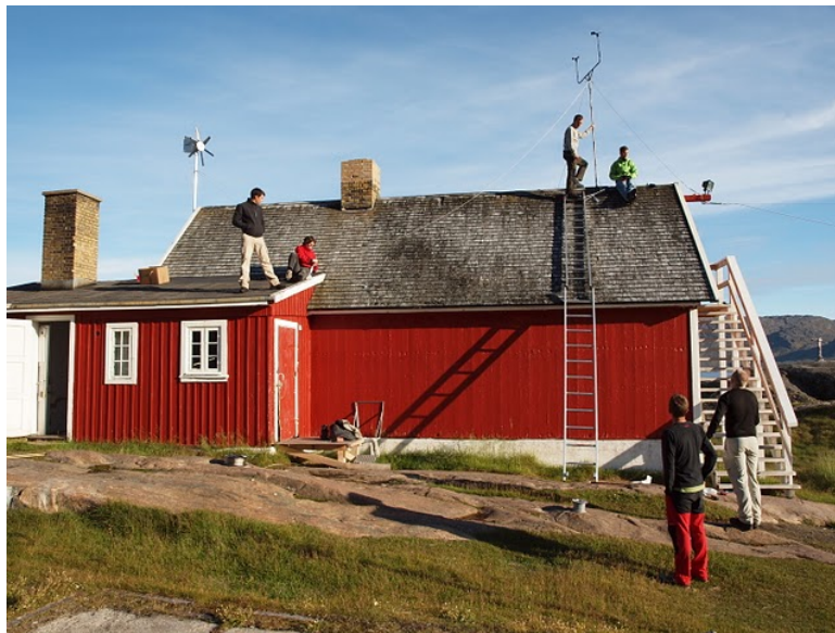
Figure 27: Installing the anemometer and wind vane.
