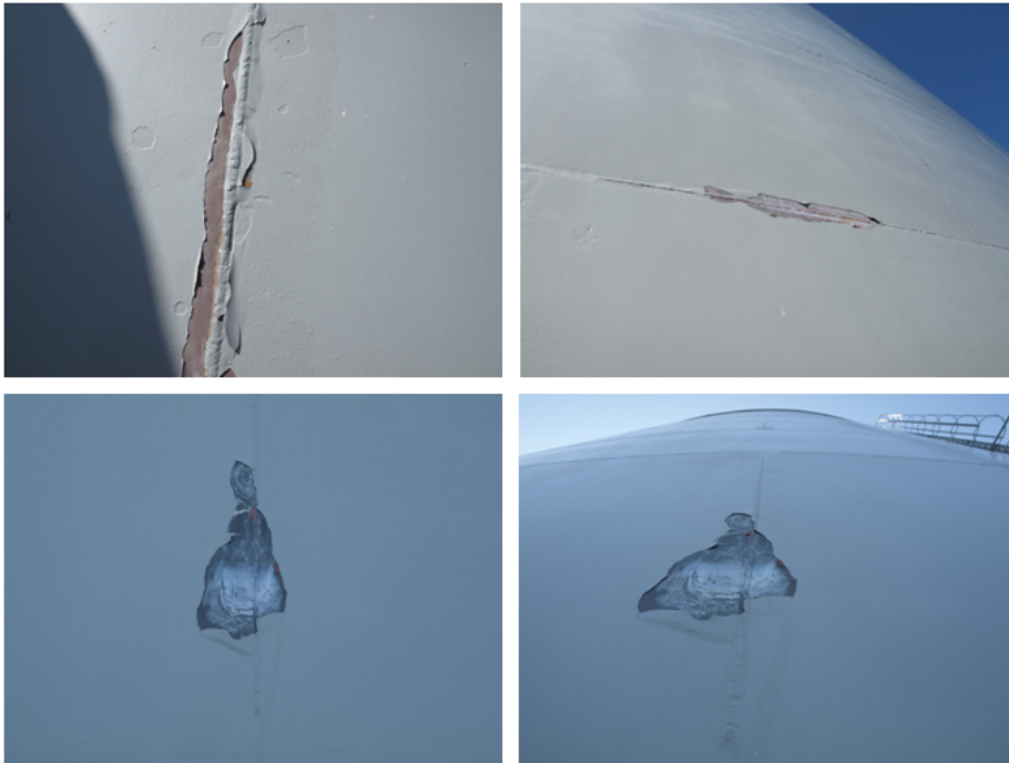
Figure 7: Stone chip damage on the tanks
